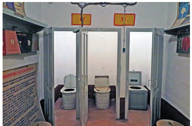
Toilets within shelter number 2. These used earth rather than a chemical solution
